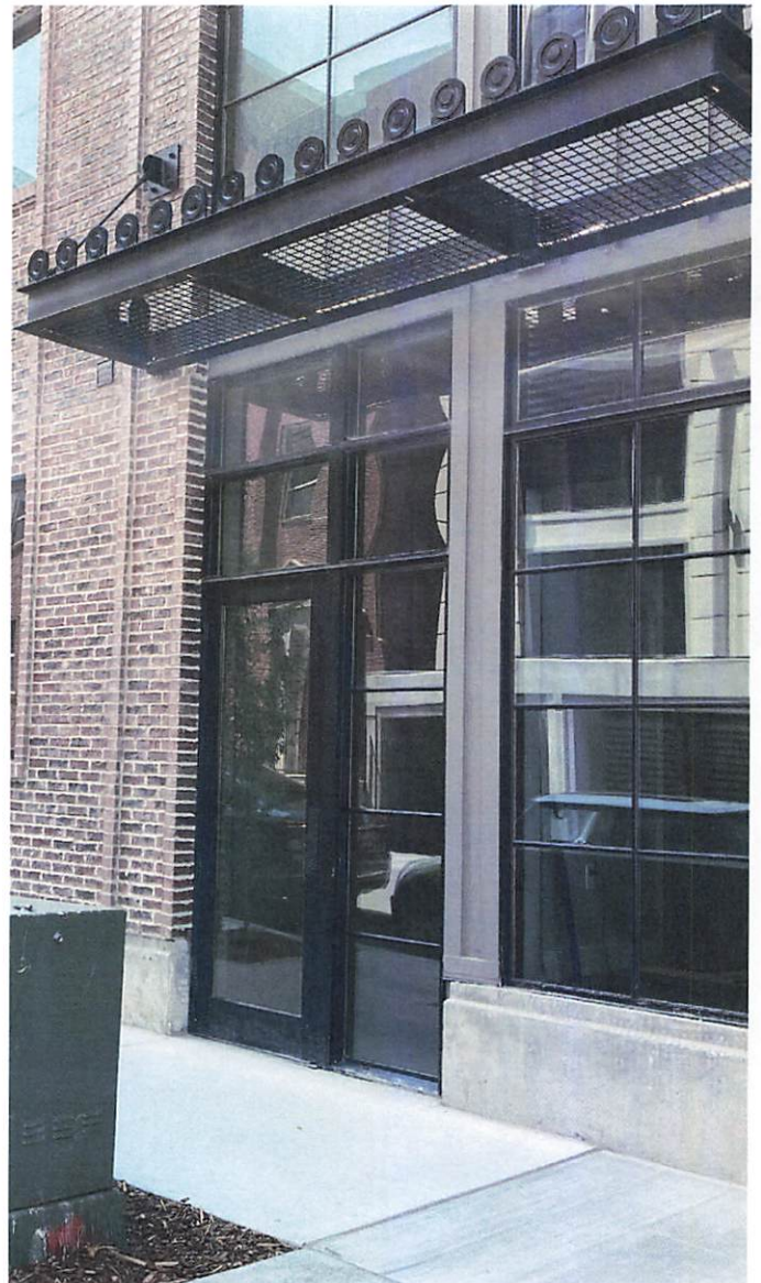
Ground floor residential units in this Salt Lake City multifamily project are tall enough that they can be converted to commercial at a later date.
