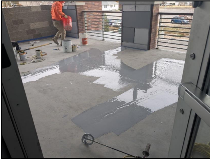
Station 81 Patio Project to Stop Leaks in Office Below
