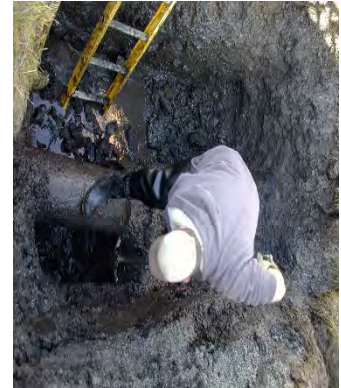
Public works repairing a leak
